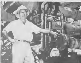
HENDRIK VAN der Kuyp, CYI suggestor-of-the-month for June, received a Fls. 690 award for his idea to install additional T-laterals on No. 3 Finger Pier.
